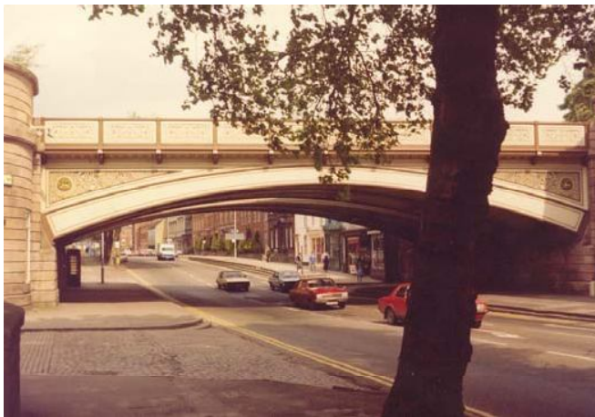
Friar Gate Bridge, Friar Gate, Derby
