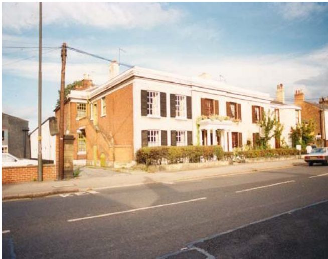
Georgian House Hotel, Friar Gate, Derby
